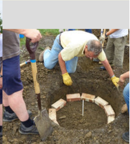
The kiln was dug out and the first course of bricks laid.
