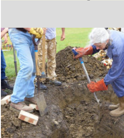
The kiln was dug out and the first course of bricks laid.
