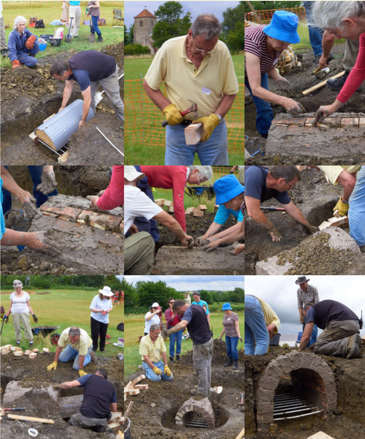
The stokehole was built and tested.
