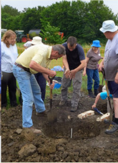
The kiln was dug out and the first course of bricks laid.
