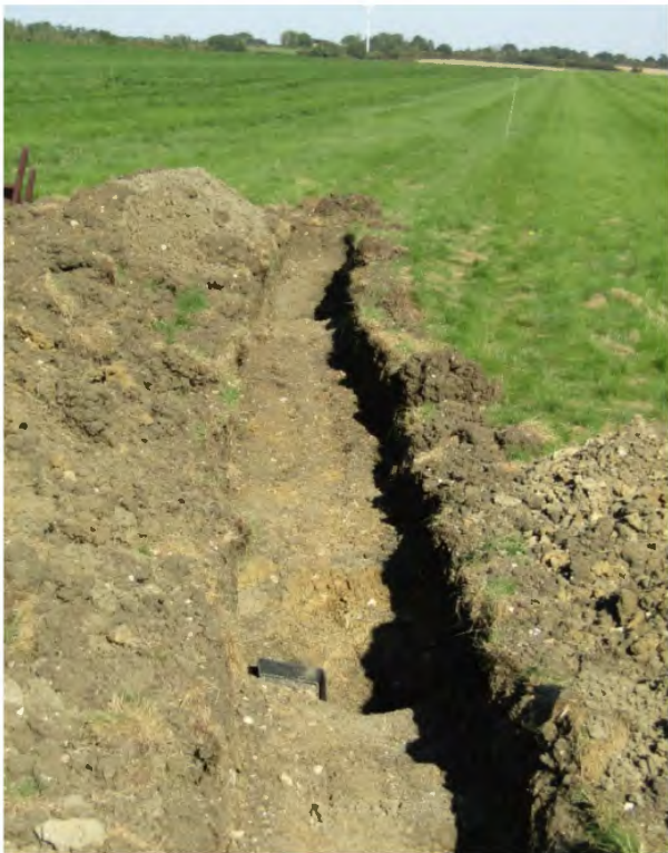
Trench 2 – Looking East
