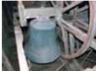
Sometime after 1600 the idea of attaching a bell to a wheel was thought of so that the bell could rotate 360 degrees. Someone then devised a Stay that stopped the bell when it reached the top of wheel so that the Ringer pulling the rope had much more control. When there was more than one bell in a tower the
